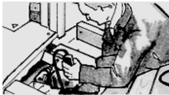
4. Using the **LARGE** holes as a guide, drill the appropriate **NUMBER** of pilot-holes in the joist, but again, **NOT** opposite each other. Use a 5mm (3/16") bit, to a depth of 30mm (1 1/4"). For 'numbers', first refer to **FIXINGS** on previous page. (Hardwood joists will require deeper holes - please consult our Technical Department).
